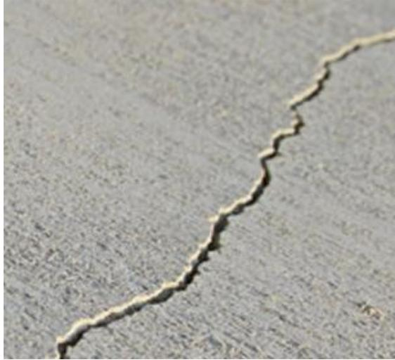
Figure 5: Drying Shrinkage Crack (SCP file photo)
