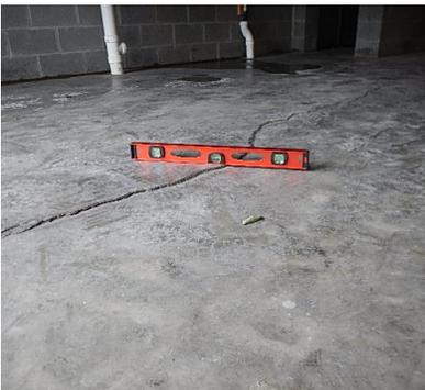
Figure 4: Settlement Cracking (SCP file photo)
