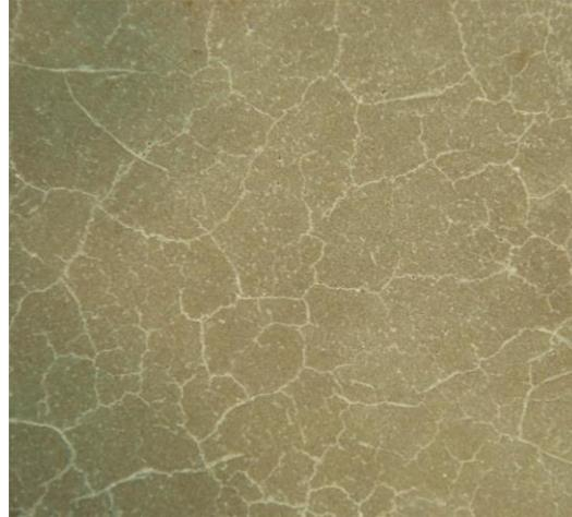
Figure 3: Crazing (image from ConcreteConstruction.net)
