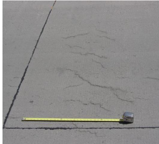
Figure 1: Plastic Shrinkage Cracks (image from ForConstructionPros.com)
